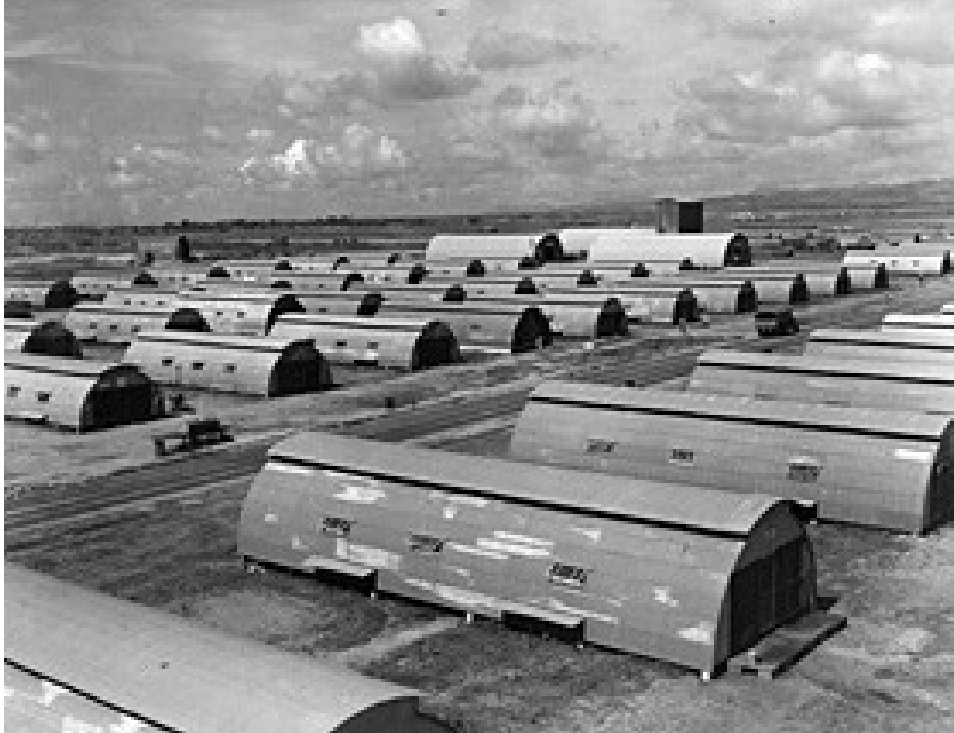
Figure 8. Stran-Steel Quonset Huts. (National Archives, RG 80-G-347017 )
