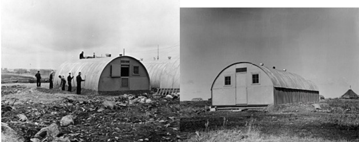
Figures 6 and 7. Original T-rib Quonset and Redesigned Quonset Huts. (National Archives -RG 80-G-7443 and RG 342-FH-3b47102)
