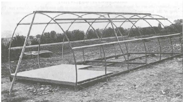
Figures 4 and 5. Wooden flooring is installed, the inner corrugated lining (horizontal) added, then the end piece and outer corrugated skin (vertical) applied. (Images from Nissens.co.uk)
