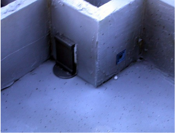
Figure 27 – Detail of a door and loophole.
